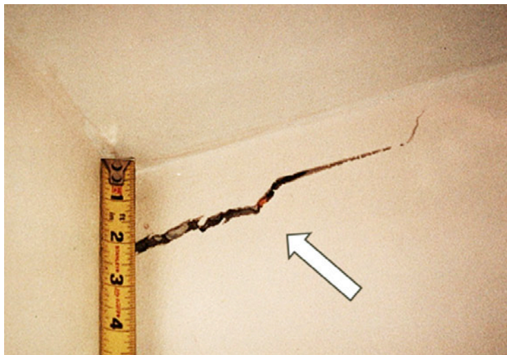
Fig. 17. Above: Burial Chamber (J), KV 62: north wall, surface relief (positive), showing diagonal separation in plastered surface. Below: Identical type of fissure as seen in a modern partition wall (Above: http://www.highres.factum-arte.org/Tutankhamun/ , detail, with additions, copyright © Factum Arte/Ministry of State for Antiquities and Heritage, Egypt, detail. Below: after http://inspectapedia.com/vision/SinkingHouse109DJFs.jpg , manipulated, with additions, copyright © InspectAPedia.com 2010)
